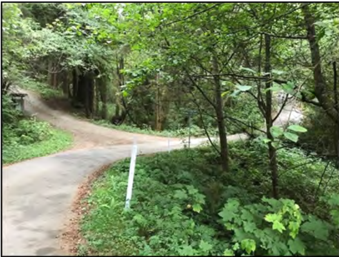
Figure 57. Flood-Prone section of Archer Road.
