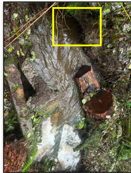
Figure 58. Duke Creek Culvert.
