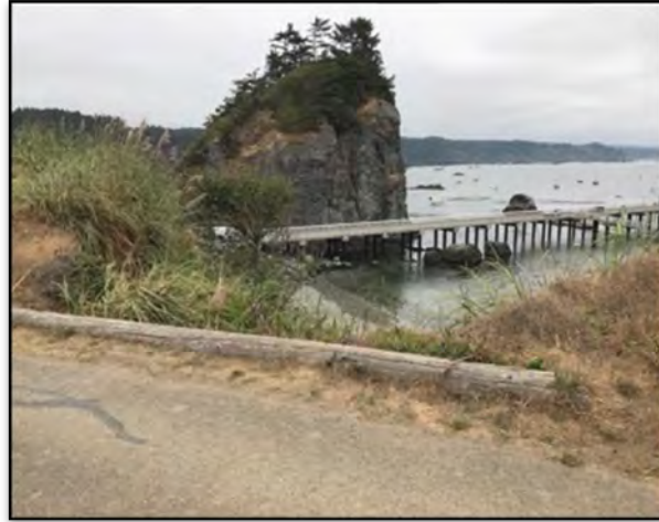
Figure 29. Erosion on Trinidad Head Access Road Next to Seascapes House.
