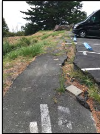
Figure 31. Erosion on Ocean Side of Heights Casino.
