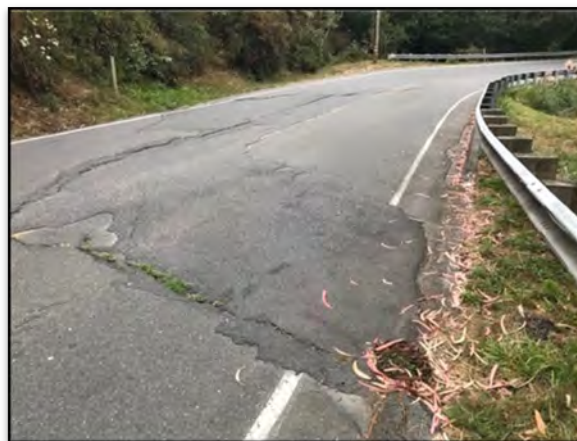
Figure 33. Scenic Drive Shoulder Erosion.
