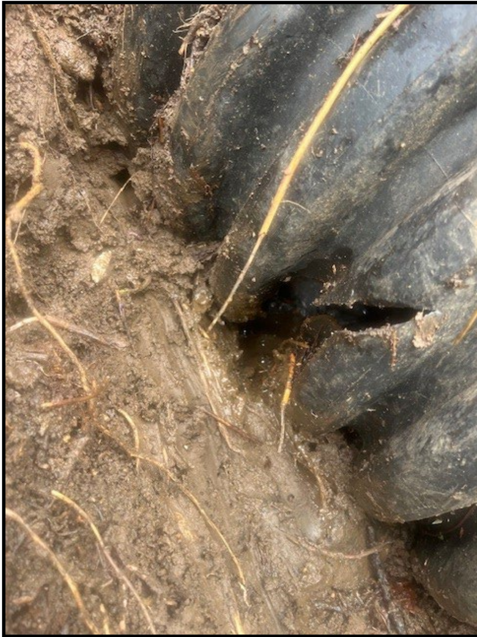
Figure 10: Exposed Pipe Going Underground with Damage Facing Towards the Parking Lot
