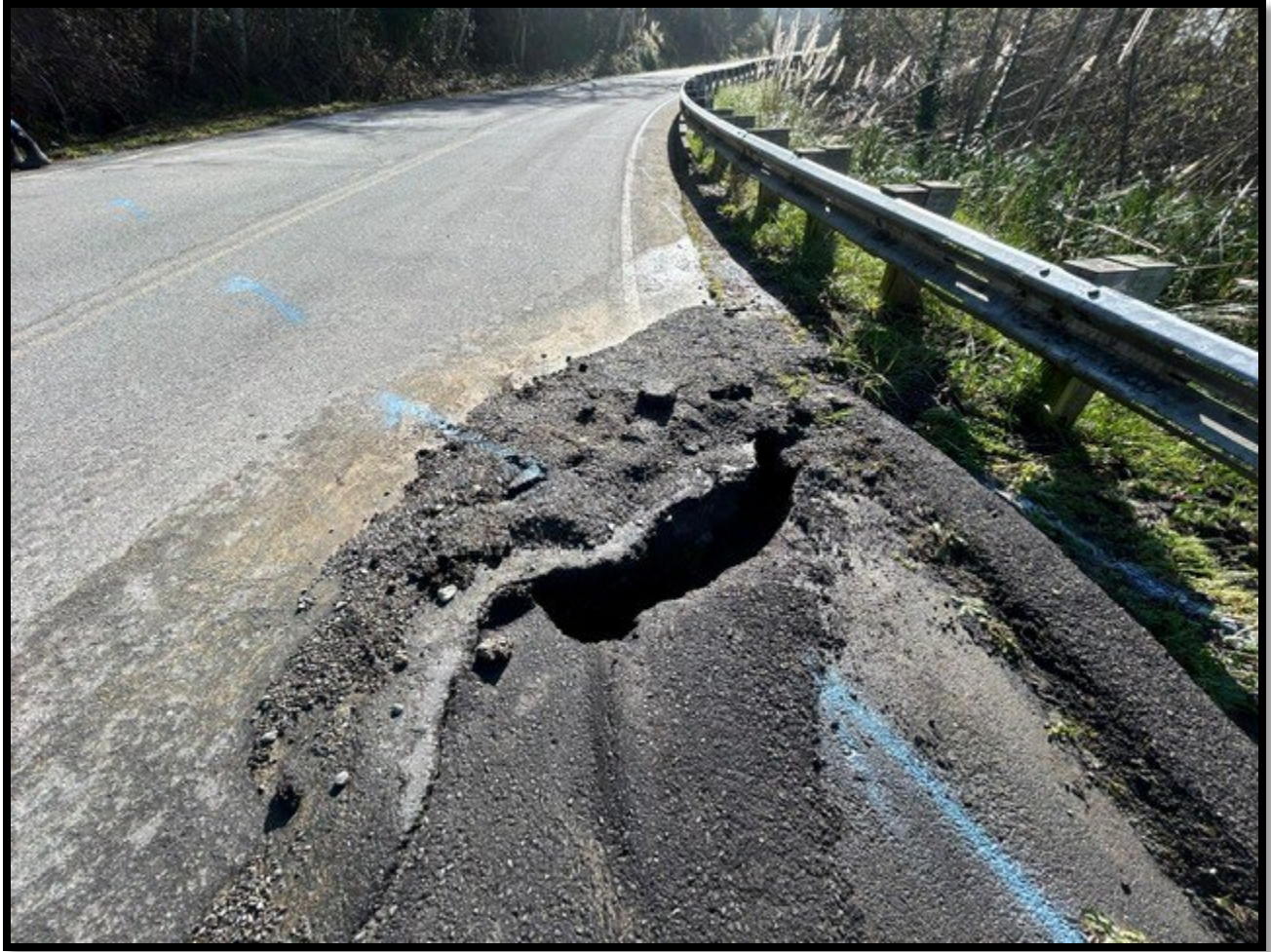
Figure 7: Road Slope Failure Due to Flooding of Site #29 Pt.2
