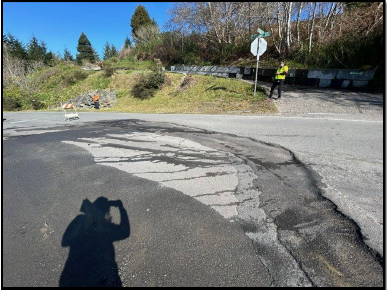
Figure 6: Road Slope Failure Due to Flooding of Site #29 Pt.1
