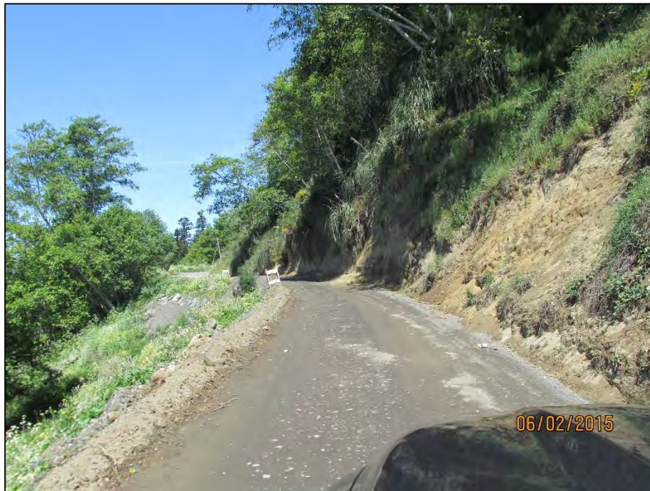
Figure 7 – Section of Scenic Drive, south of Cher-Ae Lane, showing slopes falling into Scenic Drive, and existing pavement in poor condition.
