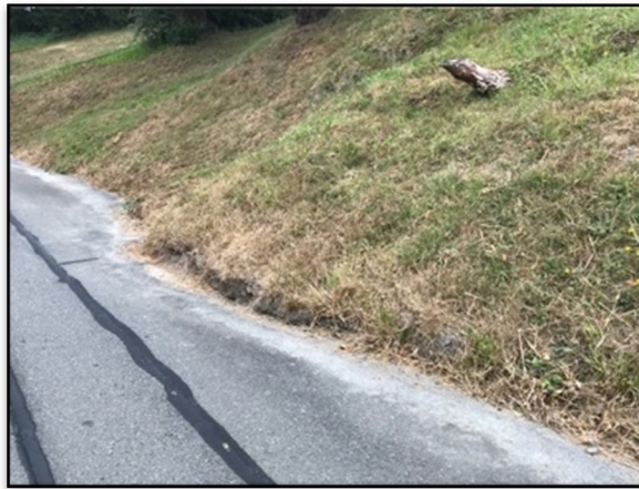
Figure 32. Erosion/slide on Cher-Ae Lane.
