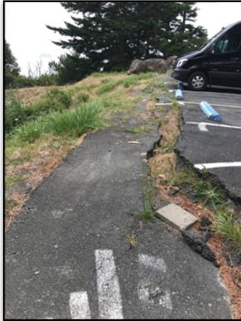
Figure 31. Erosion on Ocean Side of Heights Casino.
