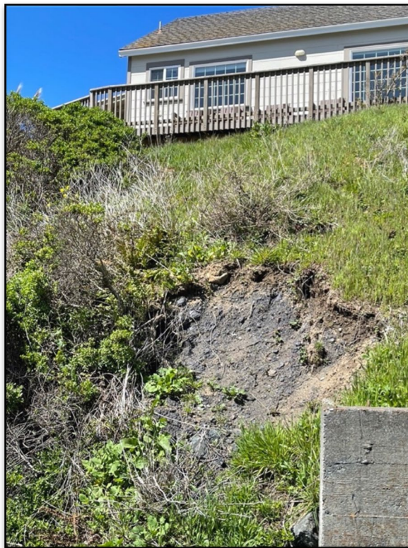
Figure 30. Erosion Below Seascape House (Trinidad Head Access Road to left).
