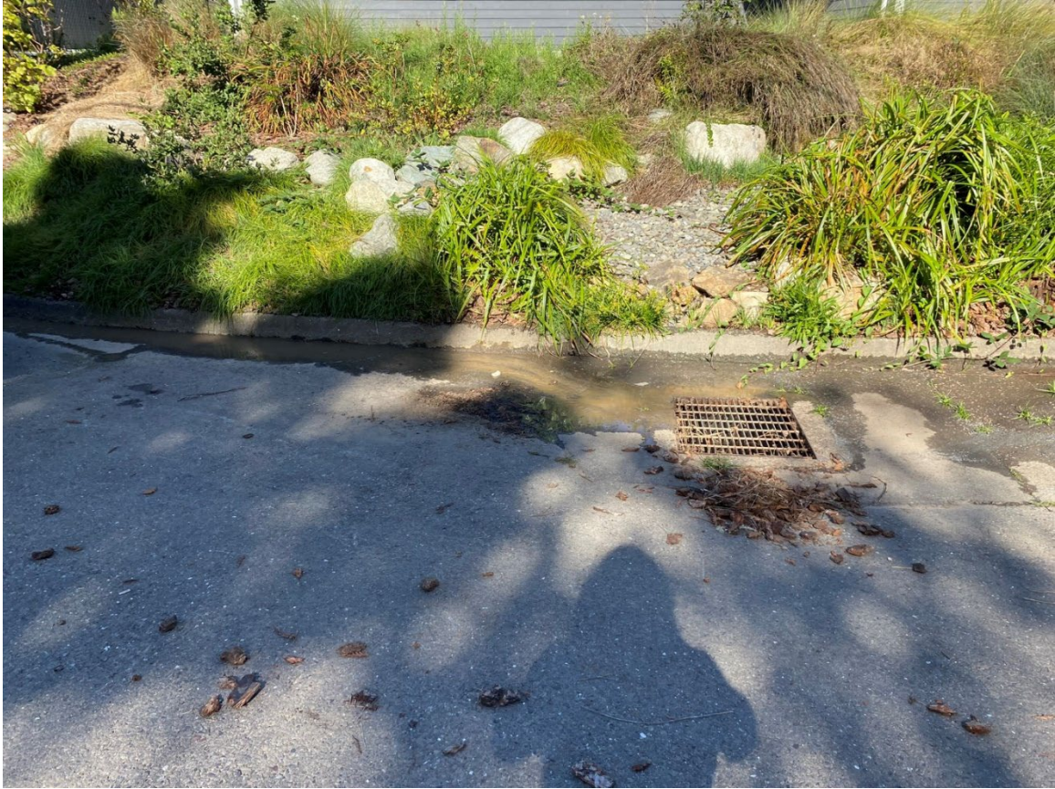
Figure 6: Inlet, North side of Ma-We-Mor View Ln
