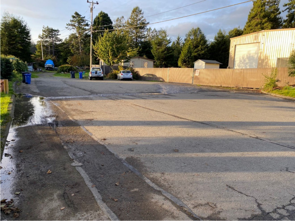
Figure 4: Contributing Drainage Area South of Inlet, Stormwater Runoff, South side of Ma-We-Mor View
